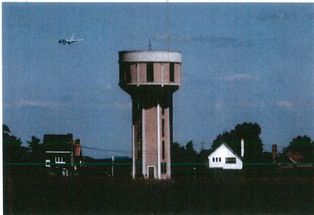
Chateau d'Eau by Bham Design Studio — Steenokkerzeel, Belgium
